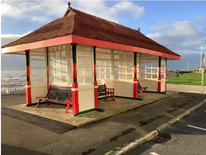
Bexhill Seafront Shelter refurbishment
