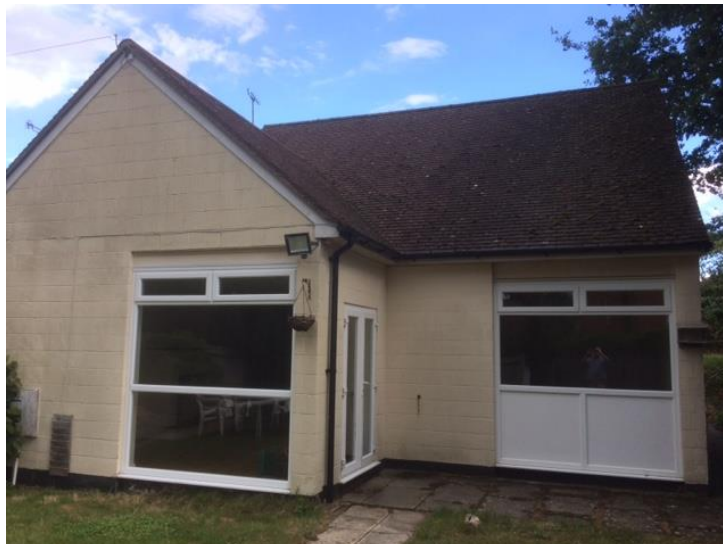
St. Francis Fields, Northiam - renovation of two bungalows in preparation for letting using CIL allocated in 2019/20
